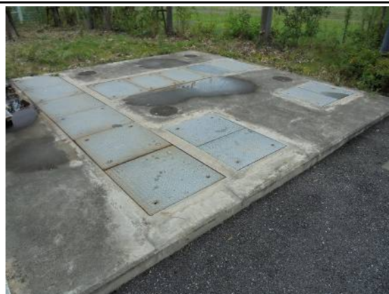
IM-3 厨房排水処理槽
